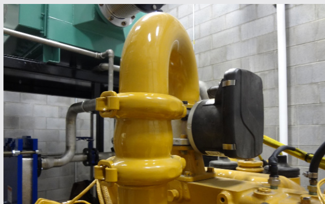
Top: TecJet 52 installed, complete with ProAct ISC actuator. Bottom: ProAct integrated throttle.
