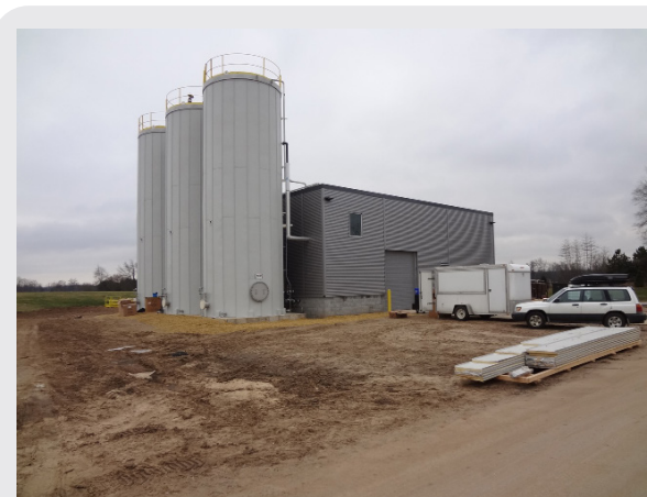
Bell's wastewater treatment plant.
