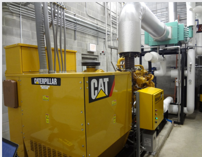
CAT G3408 genset and CHP system on-site at Bell's.
