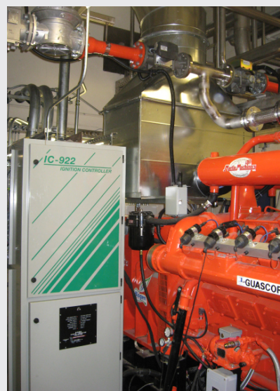
Left: Installed Woodward IC-922 Ignition Controller, Guascor SFGLD-480 V16. Right: Two angles of the TecJet gas valves installed on the SFGLD-480 V16.
