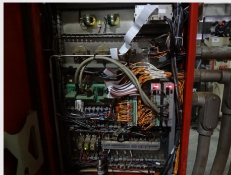
Above, left to right: Previous panel wiring and interconnections, one of four interconnected junction boxes. Below: New, simplified wiring after Woodward E6 triple stack installation.
