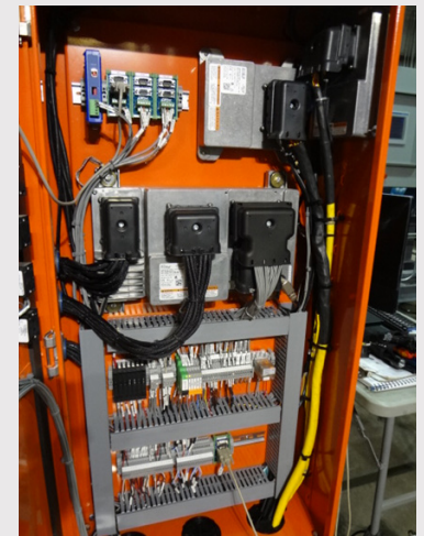
Above, left to right: Previous panel wiring and interconnections, one of four interconnected junction boxes. Below: New, simplified wiring after Woodward E6 triple stack installation.
