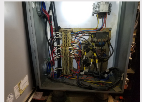
Above, left to right: Previous panel wiring and interconnections, one of four interconnected junction boxes. Below: New, simplified wiring after Woodward E6 triple stack installation.
